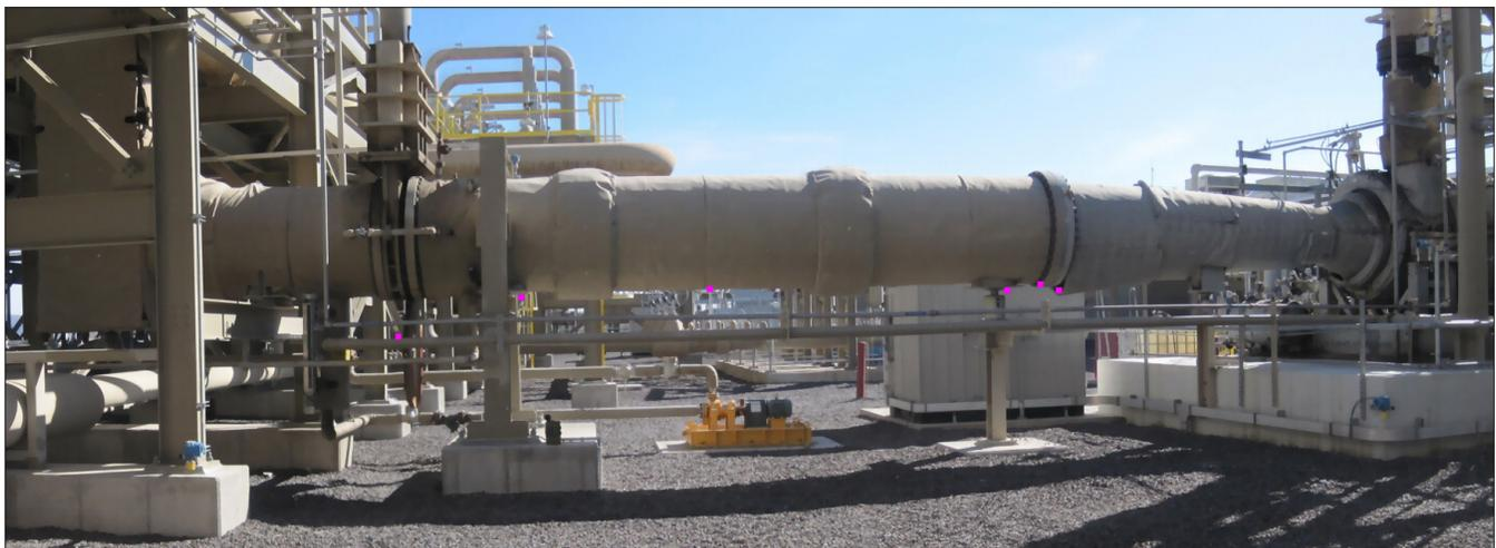
**Figure 2.** Photo of In-Service Silencer, Fully Insulated, with Turboexpander on Right Side. Flow is right to left.
