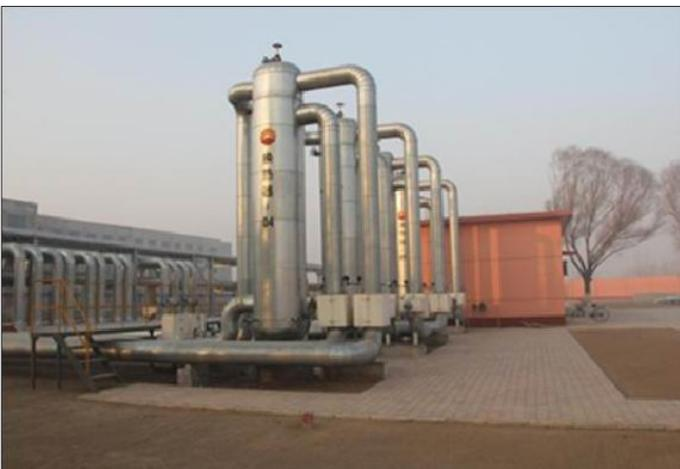
Figure 4. Heat exchanger and geothermal power generation plant.
