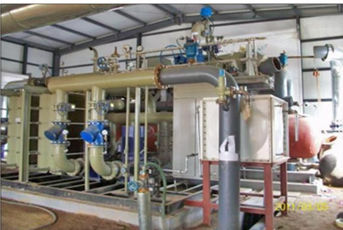
Figure 5. Geothermal power generation system: binary expander.
