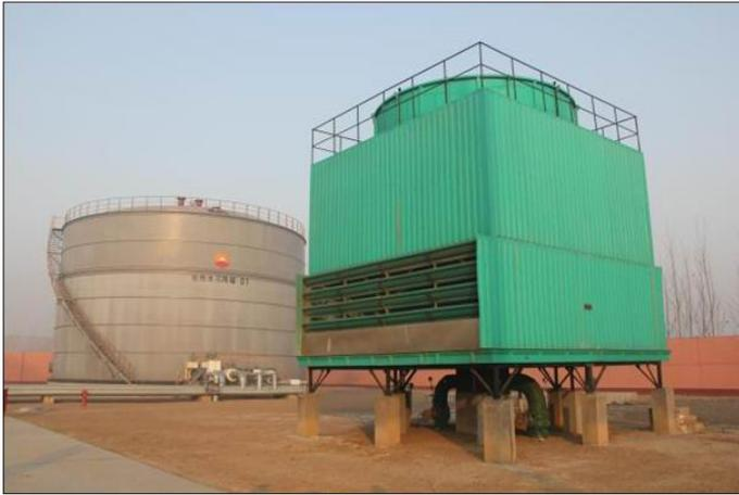
Figure 3. Oil-water tank and cooling tower.
